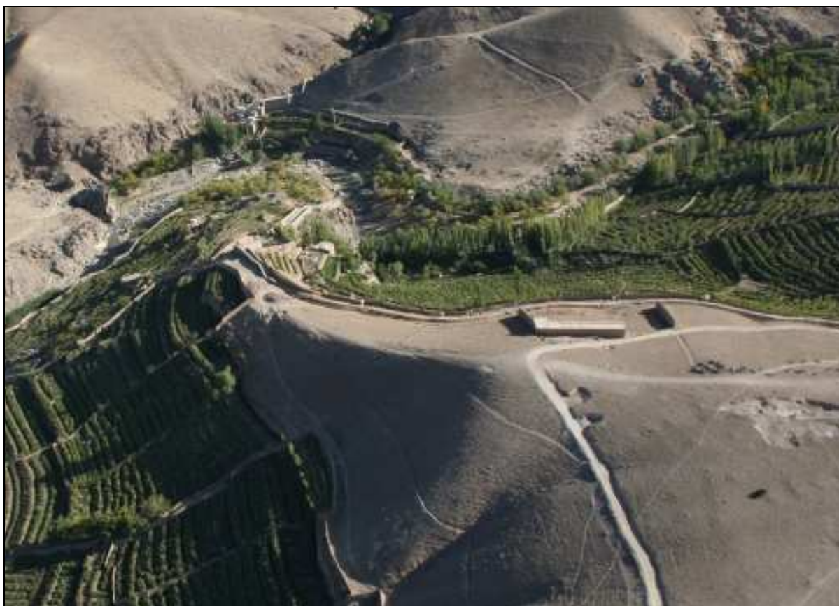
Pic.10 – View of supply channel line.
