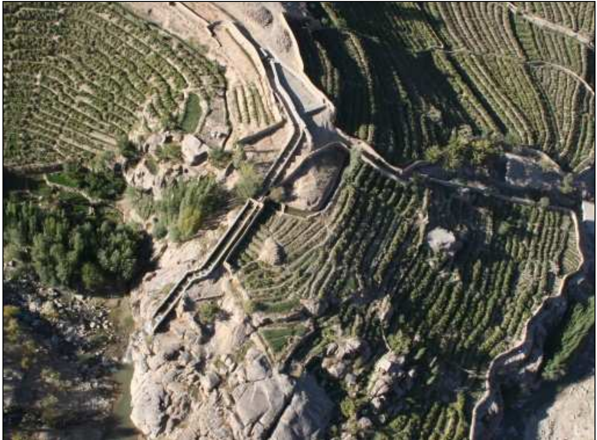
Pic.8 – Aerial photograph of the supply channel.
