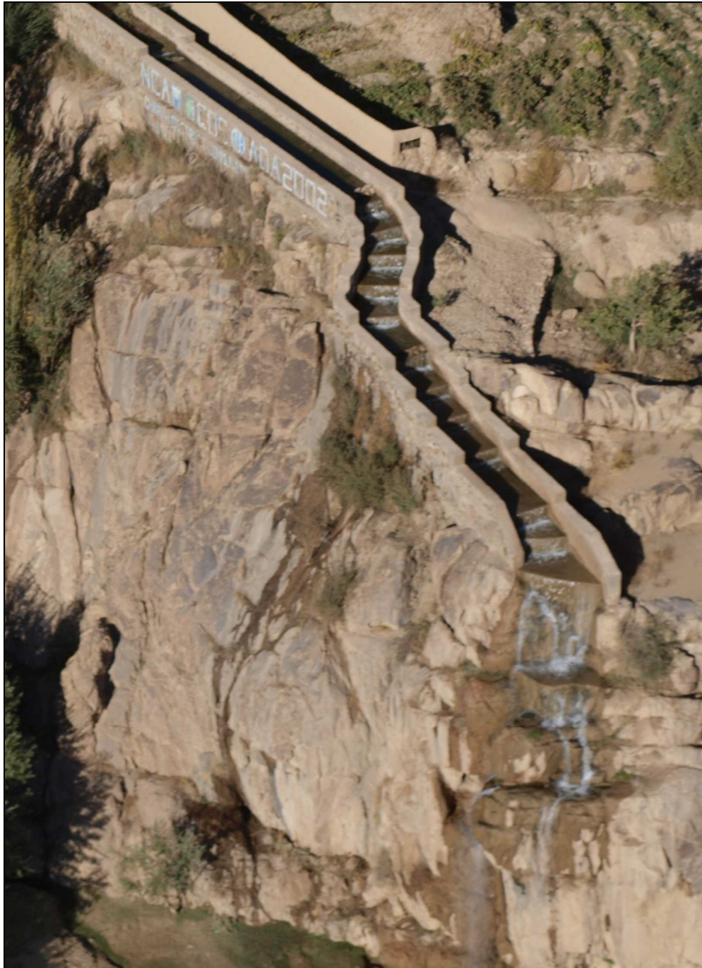
Pic.9 – Part of the unfinished micro-hydro power station.
