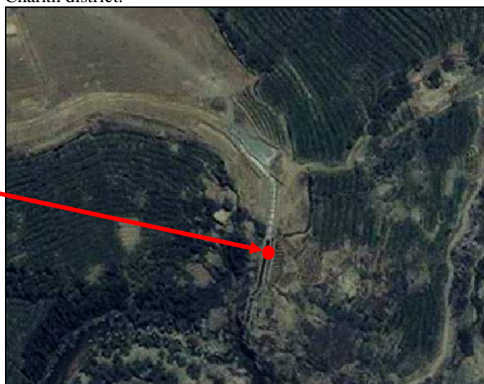
Pic.6 – satellite picture of micro-hydro power station.
