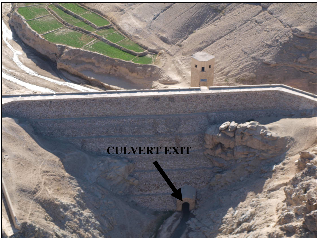
Pic.9 – Aerial photograph of air facing of the dam.
