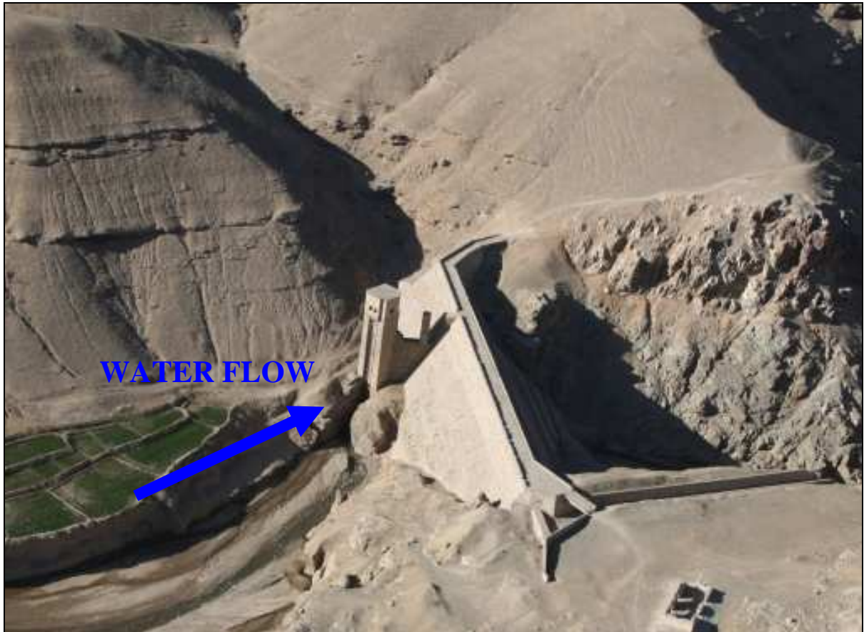
Pic.8 – Aerial photograph of water facing of the dam with control tower.
